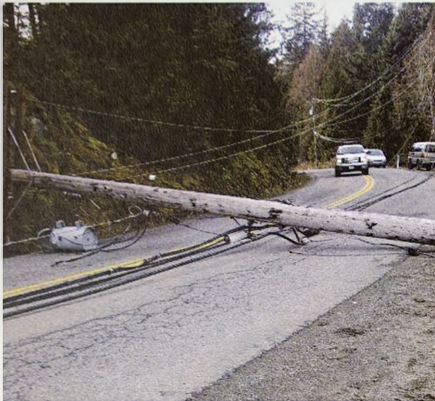
Highway 101 from Malaspina Road to Pryor Road was impassible due to downed power lines, poles and trees.
